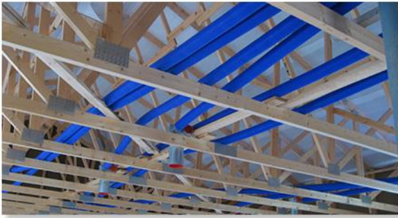
Radial ductwork Can be installed above or through eco joists
