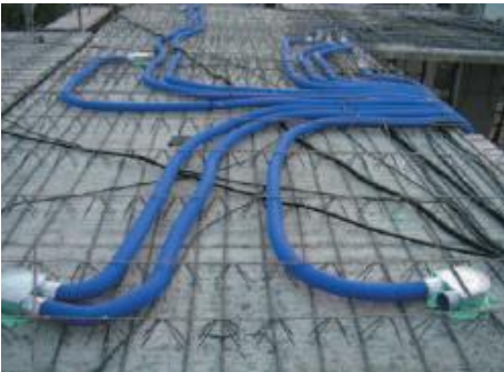
Radial ductwork Can be installed above or below a concrete ceiling
