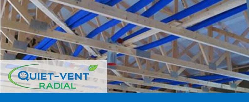
Quiet-vent Radial ducting is a crushproof, semi flexible and zero air loss system of 75mm smooth bore pipes with an antistatic and antibacterial lining individually connecting each room through a manifold.
