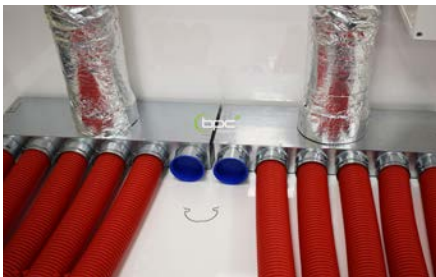
Insert the blue sealing caps as far as possible into distribution box.
