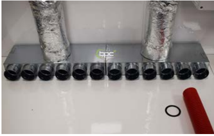
Remove pipe retaining clip from Distribution Box (if fitted).
