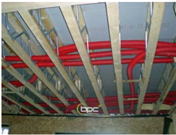
Radial duct installed through metal web joists.
