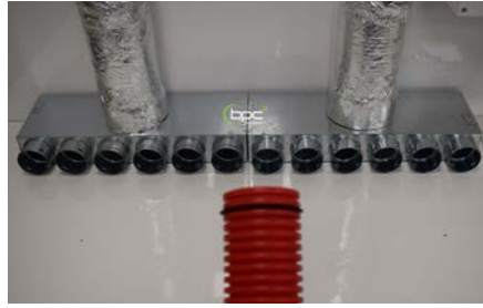
Insert sealing ring on second groove on Radial pipe.
