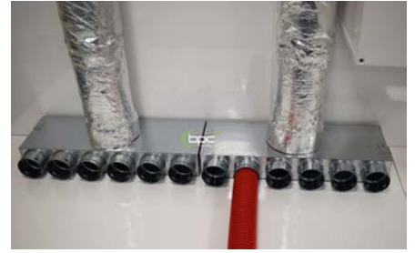
Insert pipe fully into distribution box and refit retaining clip ensuring the clip is between groove of pipe.
