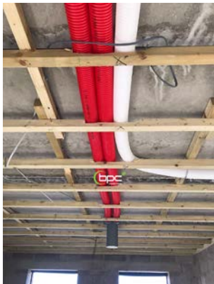
Radial pipe on concrete ceiling, allow for a 100mm crevice void.
